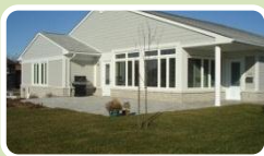
Cams Place (4 units) • North Bay
