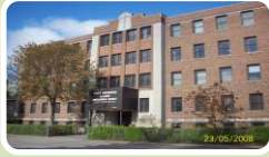
West Nipissing Centre (20 units) • Sturgeon Falls
