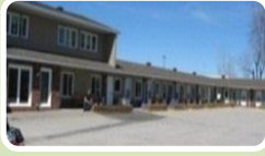
416 Lakeshore (20 units - CMHA) • North Bay
